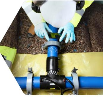
Poor installation of electrofusion fittings can result in premature leaks in water and gas distribution systems, leading to water loss, consequential damage, environmental concerns and potentially more serious health and safety considerations. JointAssist addresses this by ensuring fusion welds are completed 'right first time' from the outset by alerting or intervening to ensure critical non-conformities are not commissioned.
